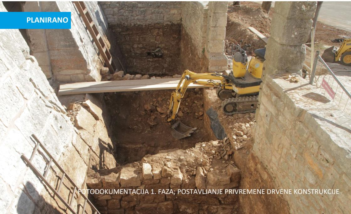
FOTODOKUMENTACIJA 1. FAZA; POSTAVLJANJE PRIVREMENE DRVNE KONSTRUKCIJE
